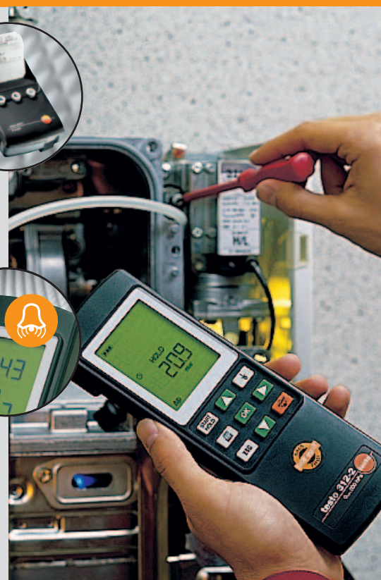
Differential pressure measurement on heating units
