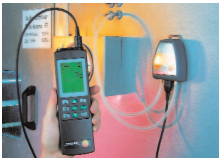
Precision meter for all pressure ranges: Differential pressure measurement at a filter with external pressure probe
